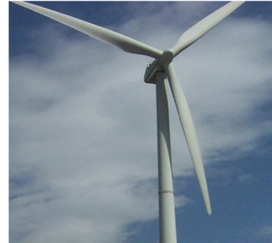
NEG Micon 750 kW wind turbine
