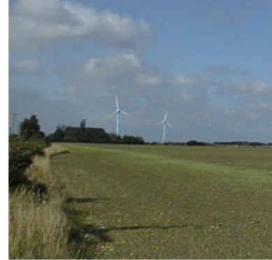
Enercon E33 WTGs at Fehmarn, Germany.
