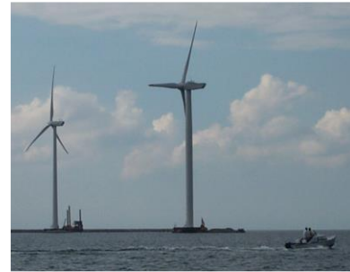
Semi-offshore turbines at Frederikshavn, Denmark.
