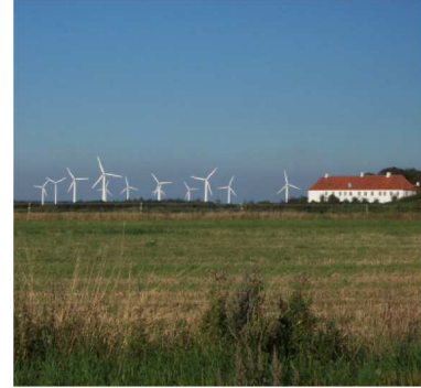
Brokilde Wind Farm
