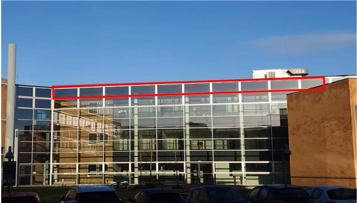
Figure 32 Windows considered in the calculation marked on a picture taken from the office
