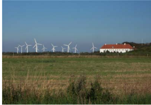
Brokilde Wind Farm, Denmark.
