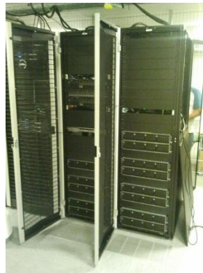
Figure 1 - Part of HPC Cluster installed at EMD
